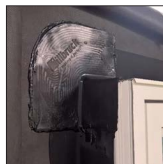
Fig 5: ME241 EPDM Corner applied to projecting window
