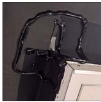
Fig 2. OT015 Adhesive beads applied; linear membrane already bonded
