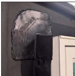
Fig 5: ME241 EPDM Corner applied to projecting window
